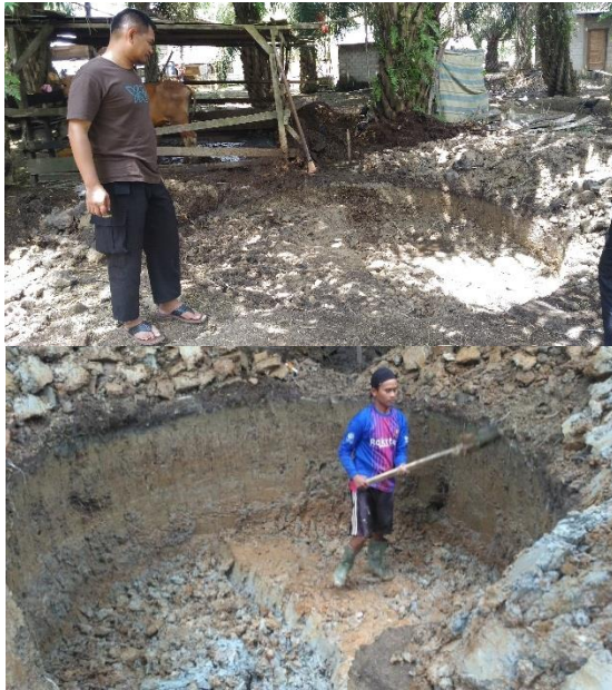
Figure 9 Digester Hole Making Process
